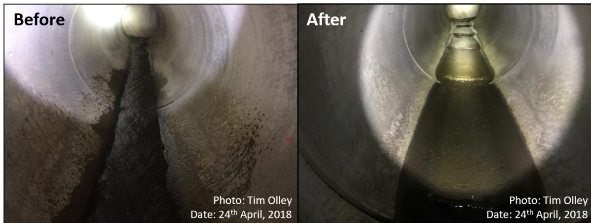
Figure 2. Lower section of the Reservoir Creek culvert before and after Flexi-baffle installation.
